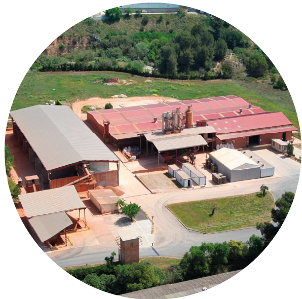
Headquarters, factory and warehouse of SIO-2 in Esparreguera (Barcelona)
